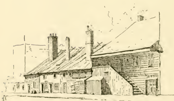
Old Houses Wiehawken St.
